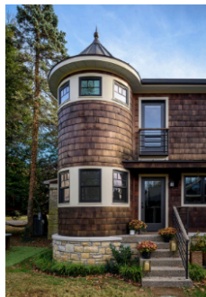
Mr. Rumancik and architect Mark Foxworth of Foxworth Architecture worked together to ensure that the turret looked like an extension of the existing architecture. They sheathed it in the same materials as the rest of the house: cedar shakes and Kentucky limestone, the latter removed and repurposed from the home’s exterior. FROM LEFT: BETHANY ADAMS; WES BATTOCLETTE FOR THE WALL STREET JOURNAL (2)
